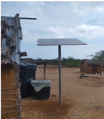
Figure 5. Installation of photovoltaic panels.
